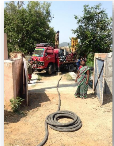
Bore well being dug at the dairy farm
